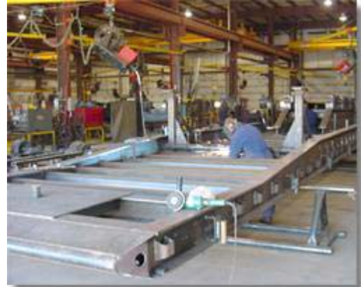
Trailer Assembly at a Scona Plant
